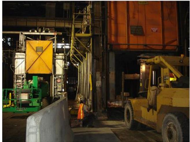
*Aligning the oven over the new foundation.*
