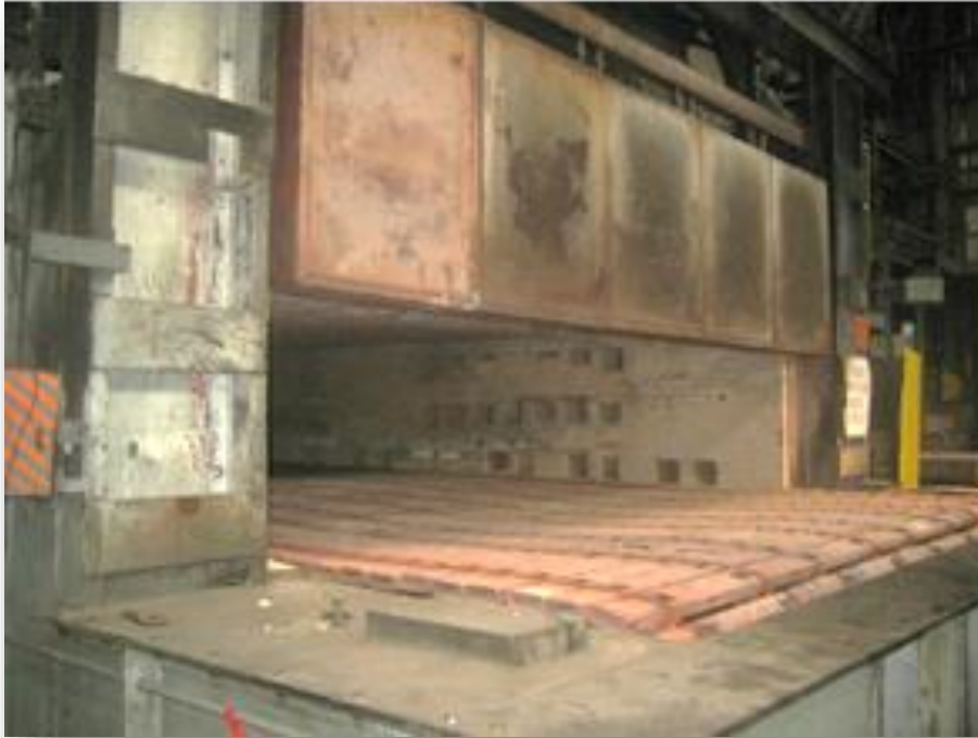
Furnace entrance before the rebuild.
